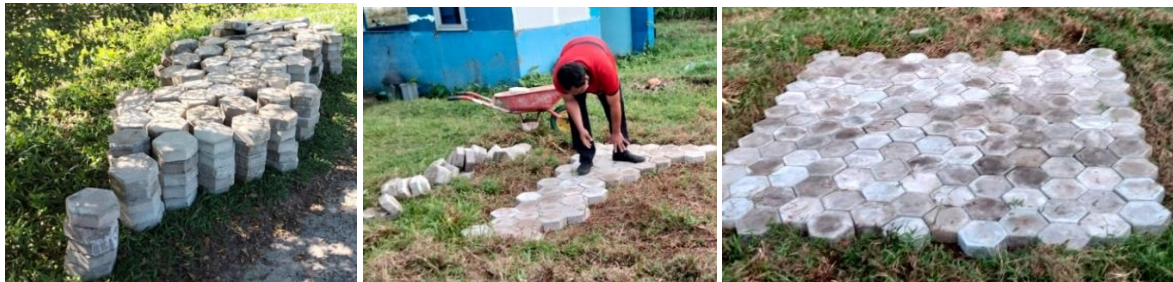
Gambar 5. Proses Pemasangan Paving Block
